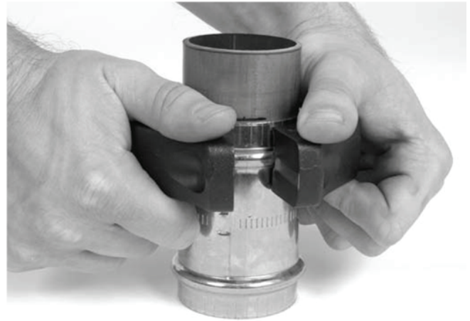
Figure 8 – Installing Press Ring Onto Fitting
